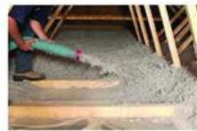
3.13 Cellulose Blown (attic)
